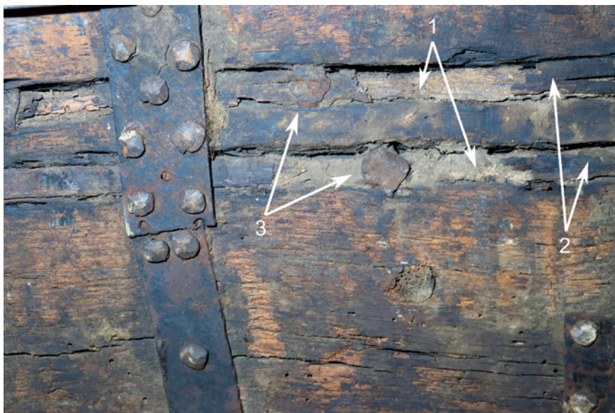
FIGURE 3 Detail of the bottom plank showing two cracks that were waterproofed with (1) moss caulking, (2) covered with a wooden lath and fastened with (3) metal sintels
