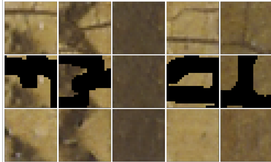
Fig 9: Example of removing detected cracks. First row: images with cracks, Second row: images with mask, Third row: removed cracks by proposed aGAN
