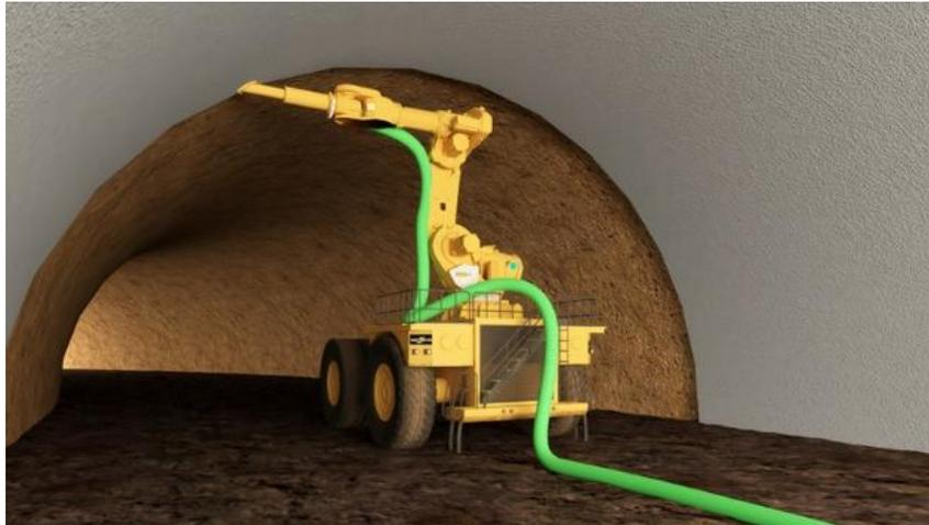
Fig. 1 Schematic view of 3D printing of a rock tunnel lining.
