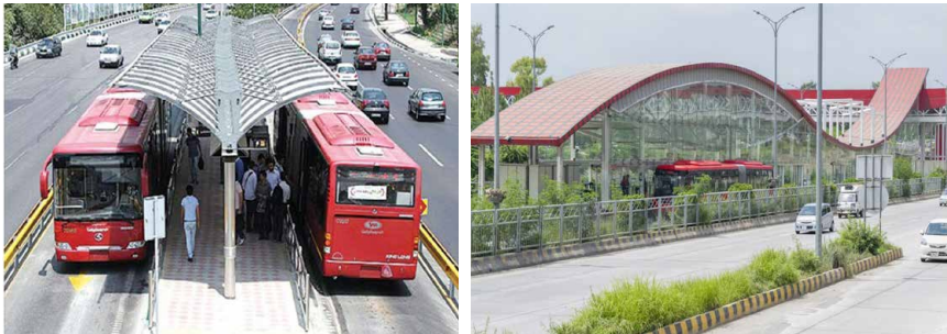
Figure 16 (a) Simple BRT station with Shelter facility (b) High-Quality BRT Station Source: (Abbas, 2018; Bajwa, 2016)
