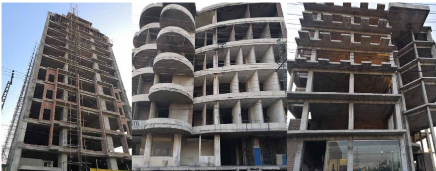
Figure 91 Under construction projects
