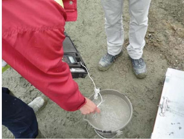
Figure 4: Temperature measurement on fresh concrete at construction site
