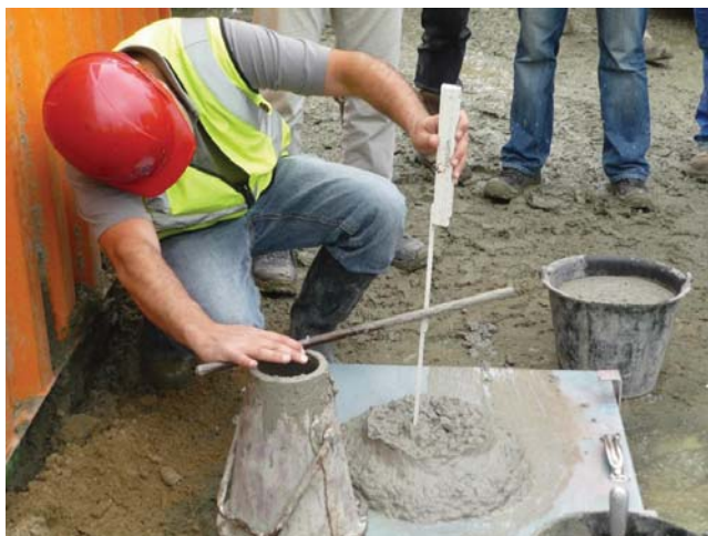
Figure 2: Slump measurement on fresh concrete at construction site
