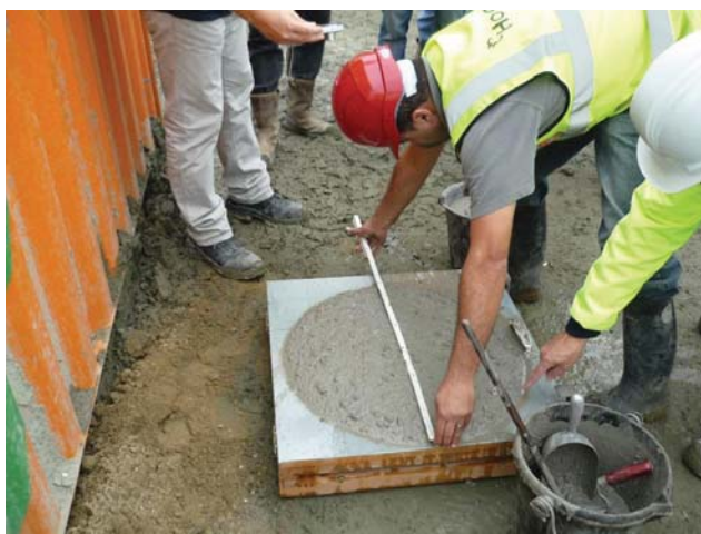
Figure 3: Flow measurement on fresh concrete at construction site
