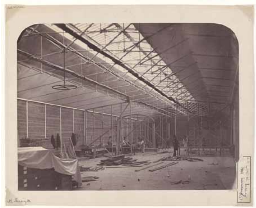
(fig. 20) Charles Thurston Thompson, Interior view of the South Kensington Museum (the 'Brompton Boilers') under construction, 1856. Architectural views of the construction of the new South Kensington Museum were taken from the start.
