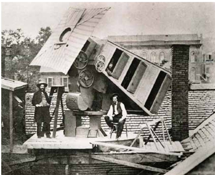
(fig. 13) The solar camera Jupiter on the roof of Van Stavoren's Nashville studio, ca. 1866.
