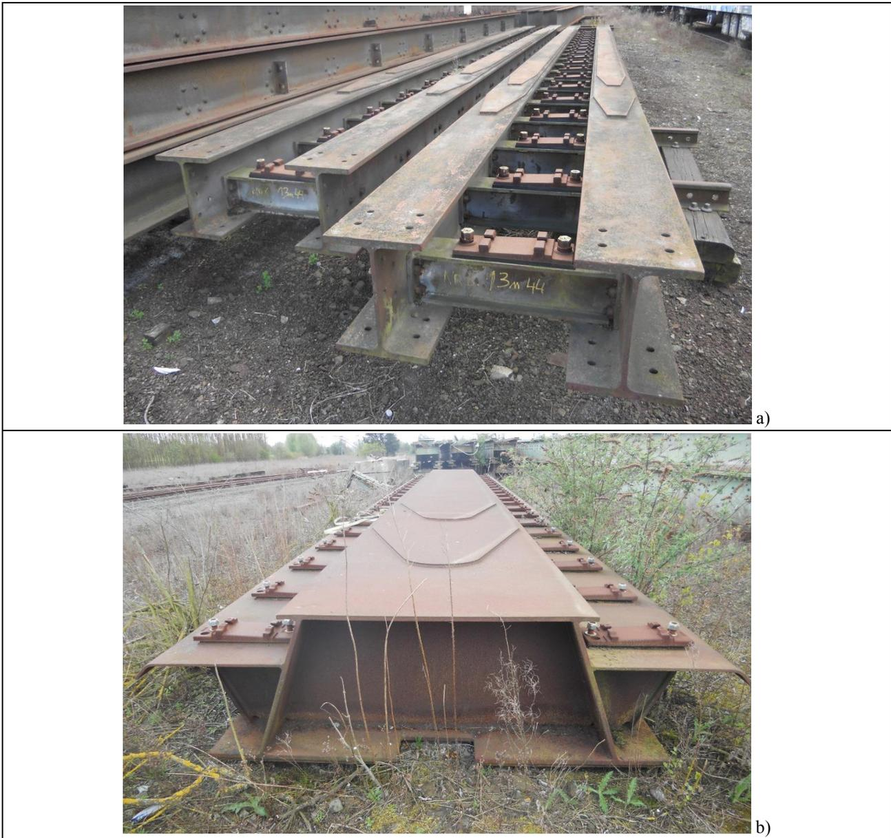
Fig. 1. a) Example of a twin girder temporary bridge deck; b) Example of a tube girder temporary bridge deck
