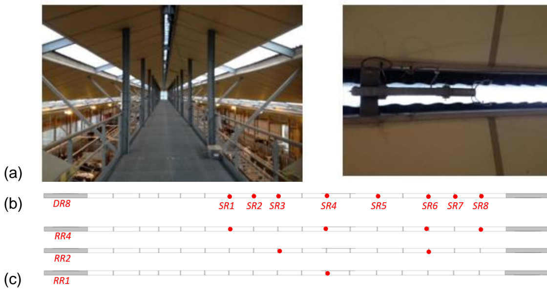
Figure 41: (a) Pictures of the bridge under the ridge vent and an example of a mounted sensor, (b) Sampling locations for the detailed measurements ridge vent ( DR8 ), (c) Reduced sampling locations ridge vent with 4, 2 and 1 locations, respectively specified as RR4 , RR2 and RR1
