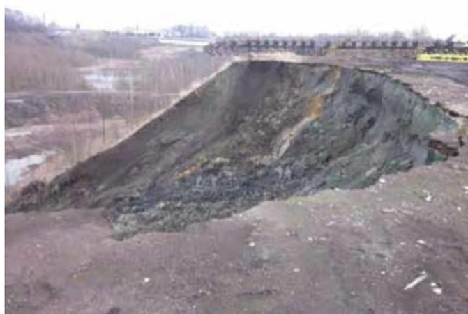
Figure 9 Photo of the unstable zone after sliding
