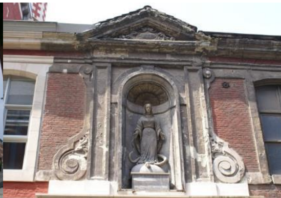
Fig. A7.4 One part of the façade is still to be restored (visible as last part of the building on Fig. 1), and the Avesnes stone is visible here. Old paint layers are visible on the stone. This is a detail of a niche on which weathering such as blistering, powdering and scaling is visible. The black deposit appears to be present on the superficial paint layer only.
