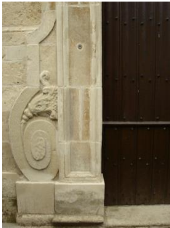
Fig. 0.1. Restoration of architectural details with repair mortar at the entrance of the St. Anne church, Bottelare, Belgium. The plinth, ornamental detail and column have been restored with repair mortar.
