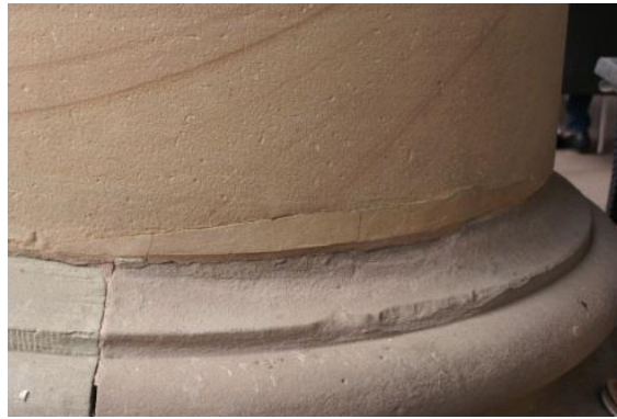
Fig. 1.1B Example of an acceptable repair mortar intervention on a column of the opera house, Strasbourg.
