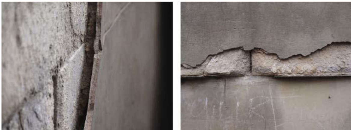
Fig. 1.3 A repair with a cement-based mortar has failed to smoothen and restore the weathered surface of these stone ashlars in Glasgow, from [12]. Both illustrations show the render loosening from the stone façade, allowing weathering of the stone beneath.
