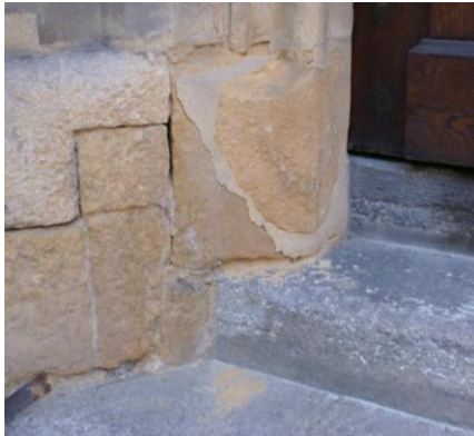
Fig. 1.1A Example of a failed repair mortar intervention on a church portico, Metz: the stone is sanding, while the mortar still appears to be in good condition.
