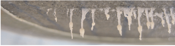
Figure 11. Formation of stalactites with a maximum height of 11 mm after a permeability test at the outlet of the crack and a crack width of 75 \mu\text{m} containing 2 m% SAP B. SAP: superabsorbent polymer.
