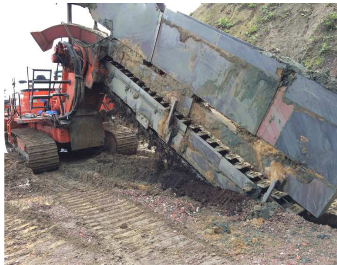
Fig. 14. Installation of the deep drainage.
