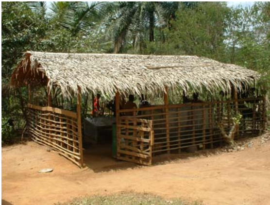
A farmer-managed vegetative propagation unit, roofed with traditional thatches in Nkom-Efoufoum, humid forest zone, Cameroon
