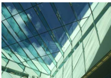
Fig. 15 - Wolfson Medical building, Glasgow
