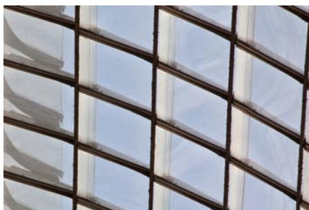
Figure 7-6: Interior view of King's Gallery of Saint-Hubertus Galleries: adjusted connection detailing after the 1993-97 restoration campaign (2010-04-22)
