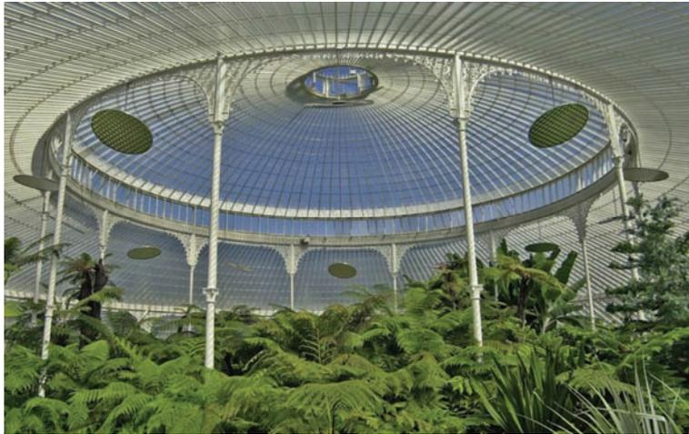
Figure 4-8: Straightened shape of main dome of Kibble Palace after 2003-06 restoration campaign<sup>51</sup>
