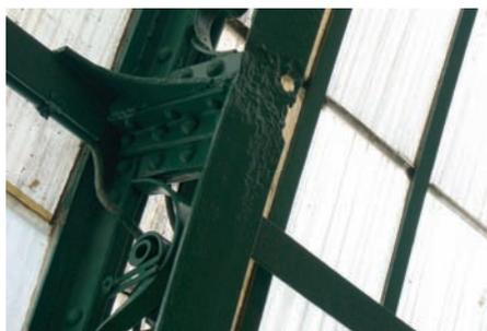
Figure 7-1: Section loss at the connection due to corrosion at the Winter Garden in Laeken (2007-03-29)
