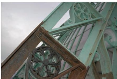
Figure 7-3: Removing paint layers at Winter Garden in Laeken (2006-11-16)
