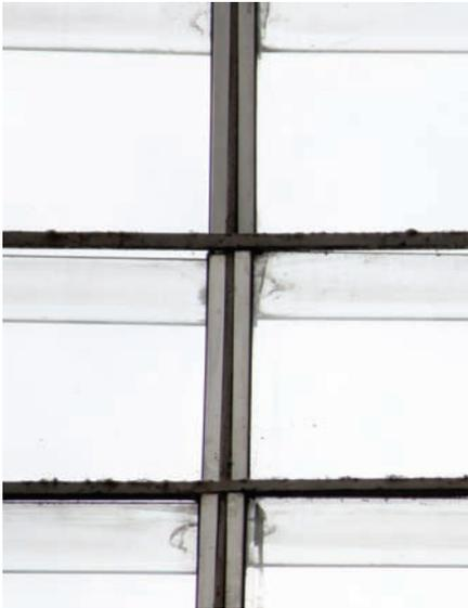
Figure 4-19: Arc with stainless-steel parclose and longitudinal L-sections after 1993-97 restoration campaign (2012-07-27)
