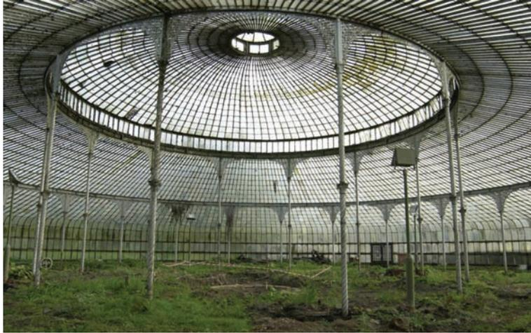
Figure 4-7: Distorted shape of main dome of Kibble Palace before 2003-06 restoration campaign<sup>50</sup>
