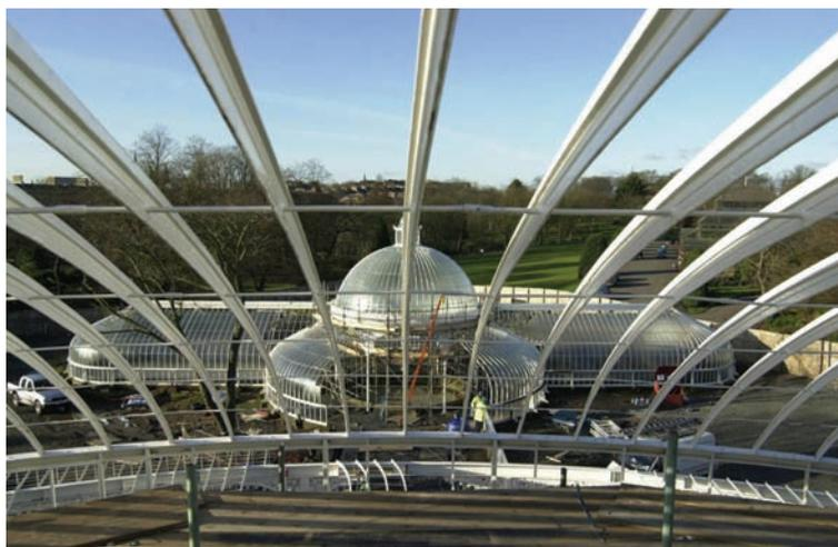
Figure 4-4: Glazing bars and ties in main dome (type c) during 2003-06 restoration campaign<sup>22</sup>
