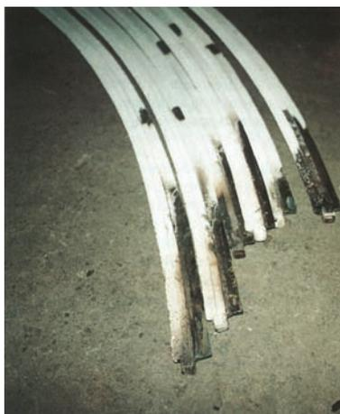
Figure 7-9: Repair of wrought-iron sections by using recycled material<sup>9</sup>
