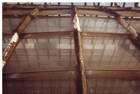
Figure 2-19: State of connections at the Saint-Hubertus Galleries before 1993-96 renovation campaign<sup>38</sup>
