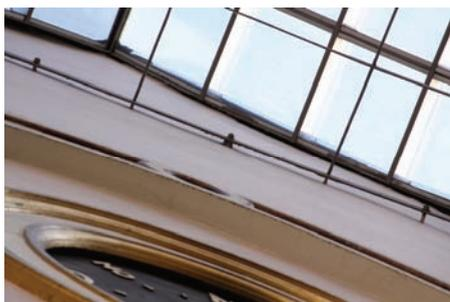
Figure 6-5: Connection of the longitudinal bars to the end walls of the galleries (2012-08-10)
