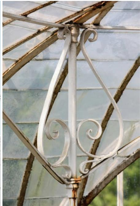
Figure 2-23: The column and its connections at the interior of the Victoria Regia Glasshouse (2010-05-20)
