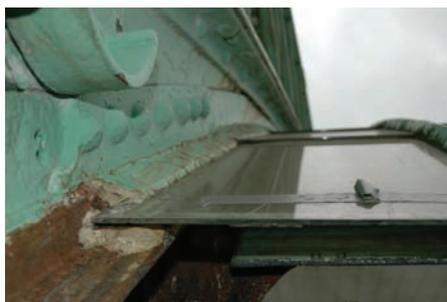
Figure 7-4: Dismantling glass plates at Winter Garden in Laeken (2006-11-16)
