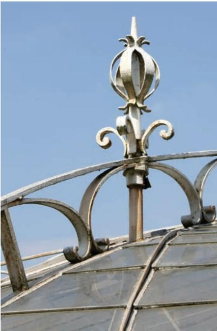
Figure 2-22: The exterior truss, the column and the triangular glass plates at the Victoria Regia Glasshouse (2010-05-20)
