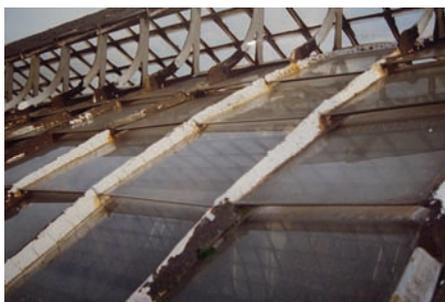
Figure 2-18: State of connections at Saint-Hubertus Galleries before 1993-96 renovation campaign<sup>37</sup>
