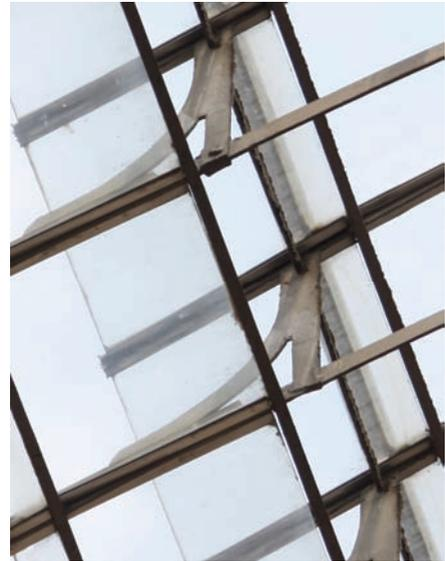
Figure 4-20: Columns between arc and lanterneau after 1993-97 restoration campaign (2012-07-27)
