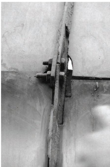
Figure 4-32: Original longitudinal connection of small roof light<sup>119</sup>
