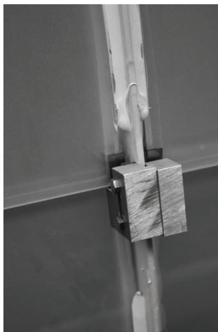
Figure 4-33: New longitudinal connection of small roof light (2010-03-02)
