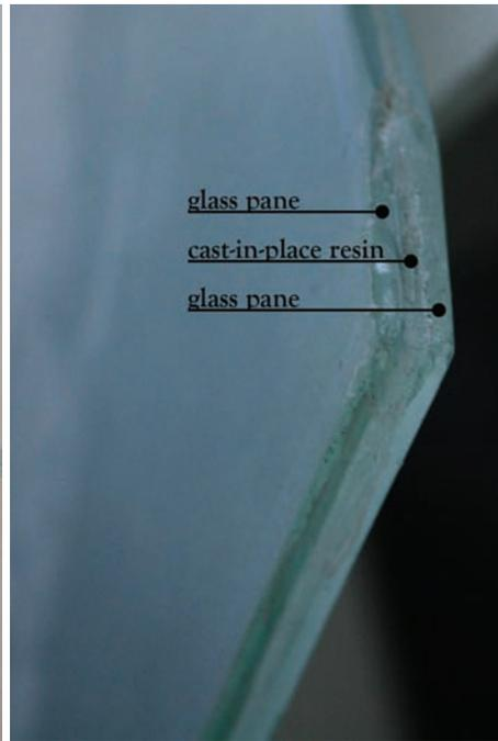
Figure 2-38: Laminated glass panels at UCB library: glass edge of cast-in-place resin laminated panel after 2003-10 renovation campaign (2010-03-02)
