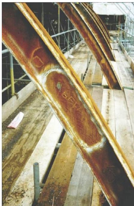
Figure 7-15: Palm House at Kew Gardens: new section in top of wrought-iron I-section<sup>14</sup>
