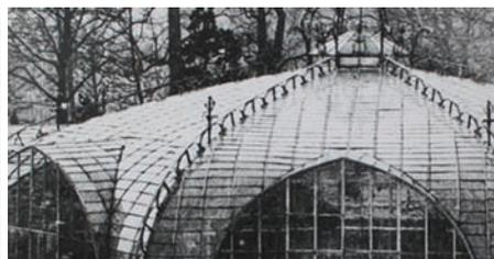
Figure 2-26: Detail of Victoria Regia Glasshouse in 1910: small glass plates<sup>42</sup>
