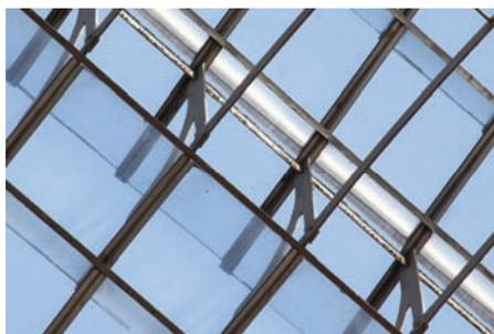
Figure 6-6: Interior view of connections between iron components: columns connected to the arcs, longitudinal column plates to the columns, longitudinal L-sections to the arches (2011-09-17)
