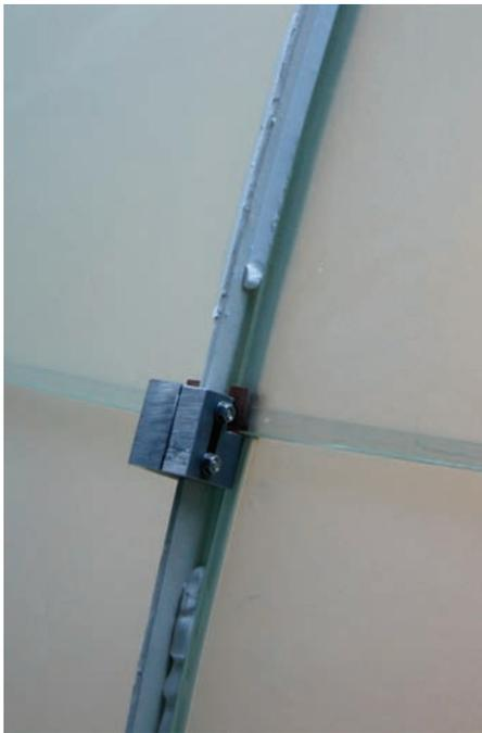
Figure 2-37: Longitudinal connection at UCB library: adjusted connection after 2003-10 renovation campaign (2010-03-02)
