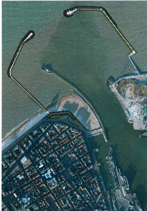
Figure 2. Renewed harbour entrance, protected by the Eastern and Western breakwaters (to be finished by august 2012)
