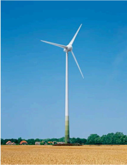
Figuur 3: 3-bladige windturbine met horizontale as
