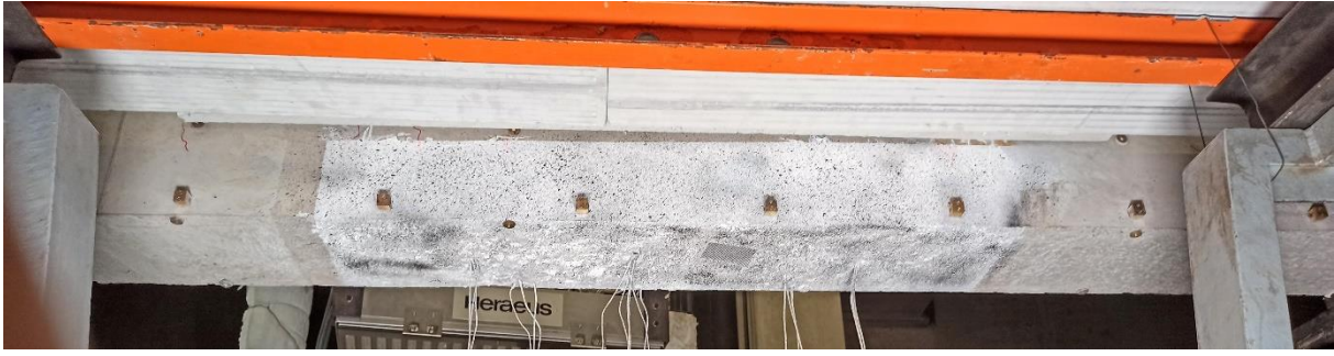
Figure 4. The compressed side of the beams monitored using the Digital Image Correlation (DIC).
