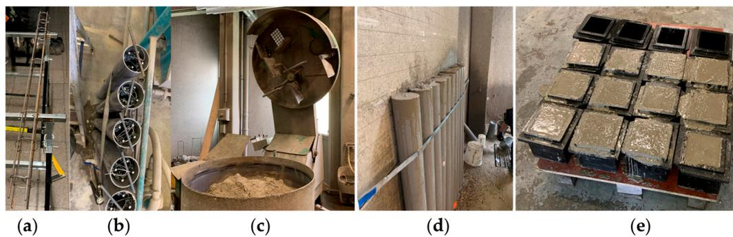
**Figure 4.** Column casting process: (a) preparation of the reinforcement cage, (b) preparation of the formwork, (c) mixture of the concrete components, (d) column pouring and (e) concrete block pouring.
