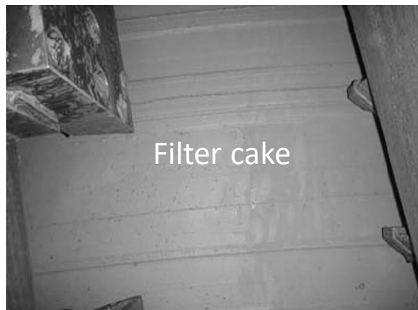
Fig. 1. Filter cake formed on the tunnel face during hyperbaric intervention in the Nanjing Yangtze River Tunnel (modified after Zhu et al., 2019)
